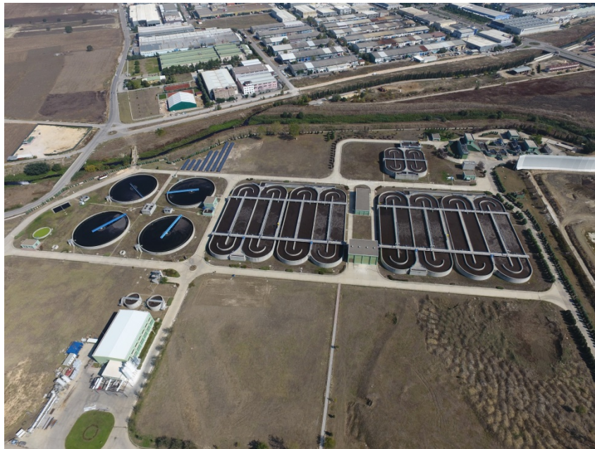
Example of Sewage Disposal (Bursa Uludag University, Turkey) : Wastewater treatment plant of the city that receives the sewage generated by Bursa Uludag University
