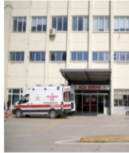
Entrance of the Emergency Room
