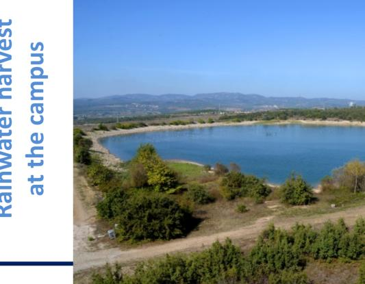
**Bursa Uludag University pond was** constructed in 2002. The volume of the pond is 0.69 hm<sup>3</sup>. The pond serves irrigational purposes within the main campus. All of the gardens and arable fields within the campus are irrigated using the water in the pond. The pond harvests rainwater.
