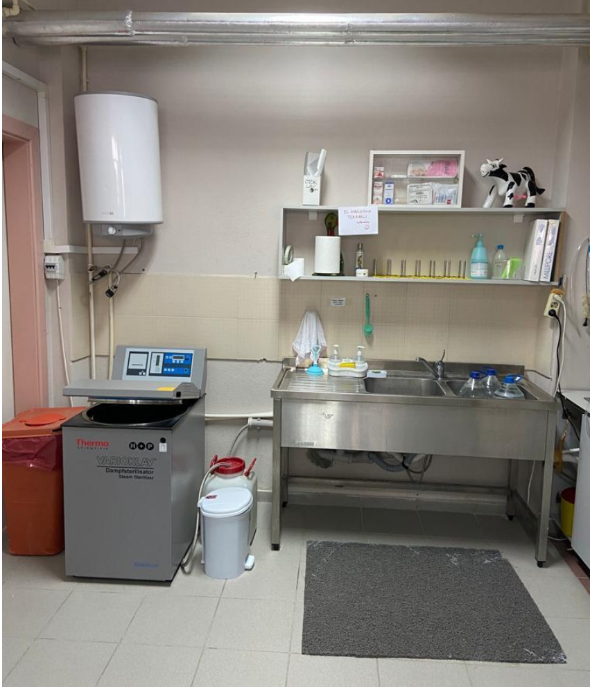
Sterilization Unit and Cleaning Area
